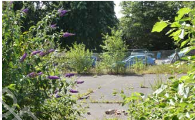
Picture of former school concrete pad and School Lane school drop-off parking
